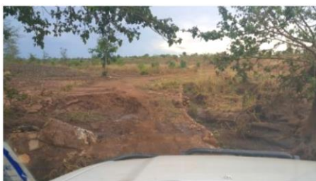
The damaged bridge close to the orphanage
